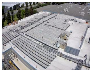
For California Dairies (USA) process heat for a dairy factory
