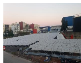
For Shell-Vivo (MO) process steam for a lubricant facility
