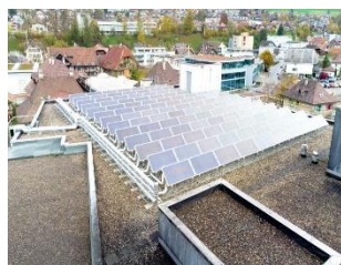
For EMMI (CH) process heat for a dairy factory
