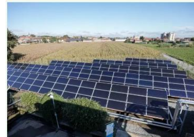
For ENGIE in Racconigi (IT) serving the largest DH operator worldwide
